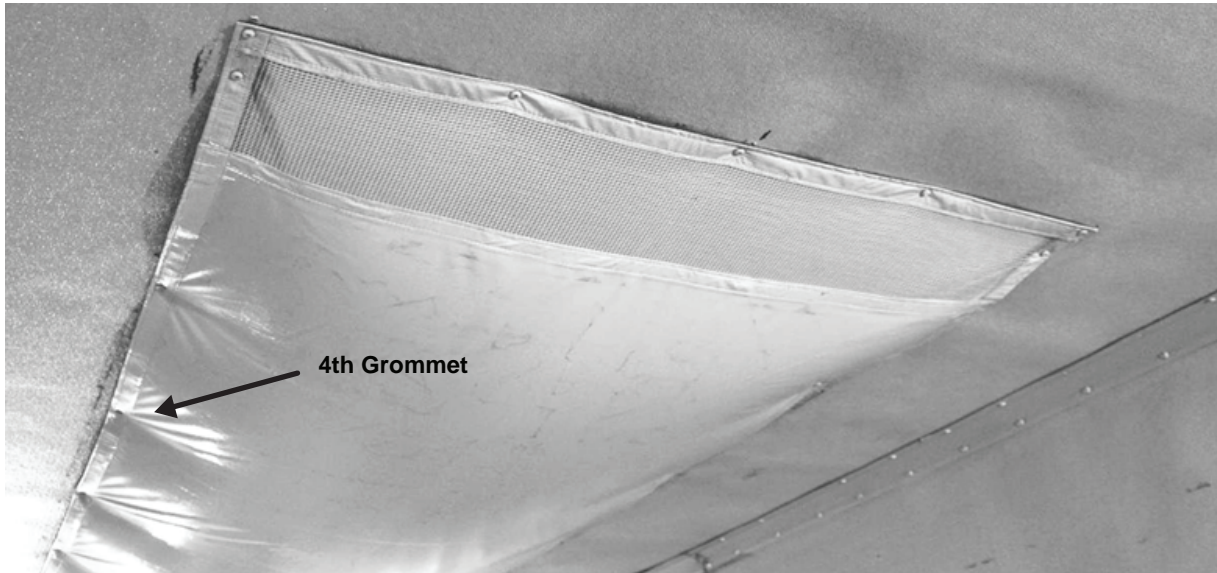
Figure 5. End of air chute shown installed flat and properly secured.
