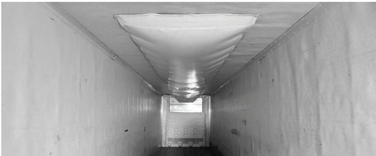
Figure 6. Completed air chute installation shown.
