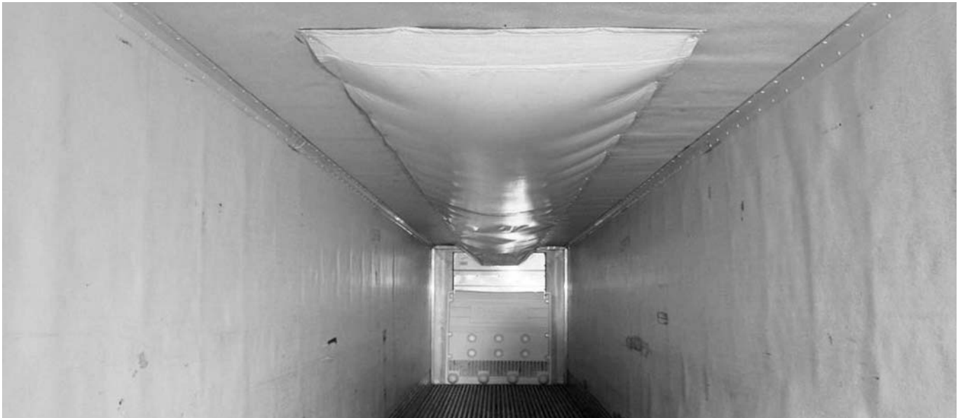
Figure 6: Completed air chute installation shown.
