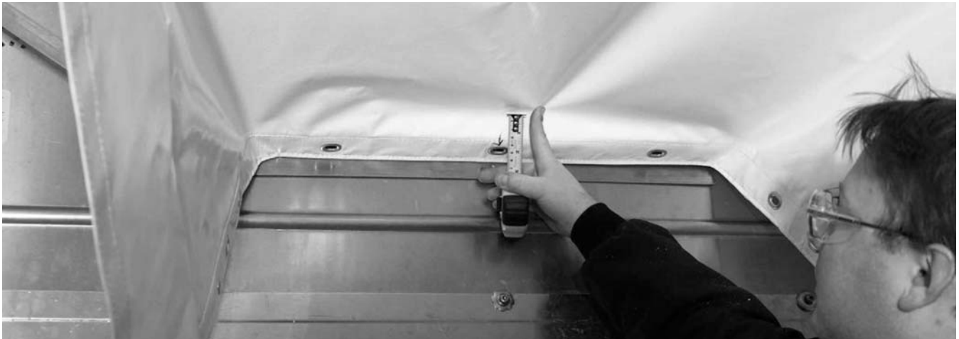
Figure 2: Chute slack in front of air outlet should be 1.00 in. to 2.00 in.
