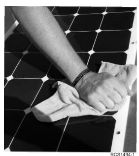
Figure 4. Firmly press panel down over entire area
